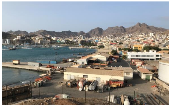
D. Potentially good as a supplementary photo if the site in the foreground represents an important aspect of the area. But it impossible to tell if the city in the background is poor or wealthy.
